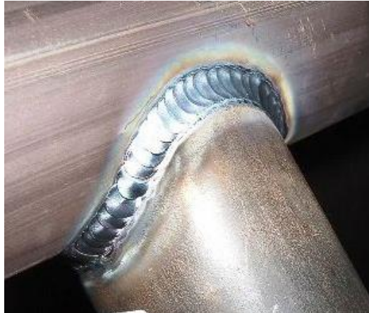
Figure 4.1: Welding of a tubular connection ( https://www.i depot.ie/blog/inverter-welder/ ).
